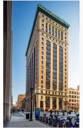
315 Park Avenue South
