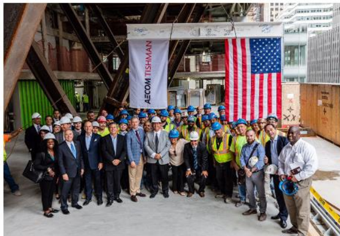
390 Madison Avenue topping out.
