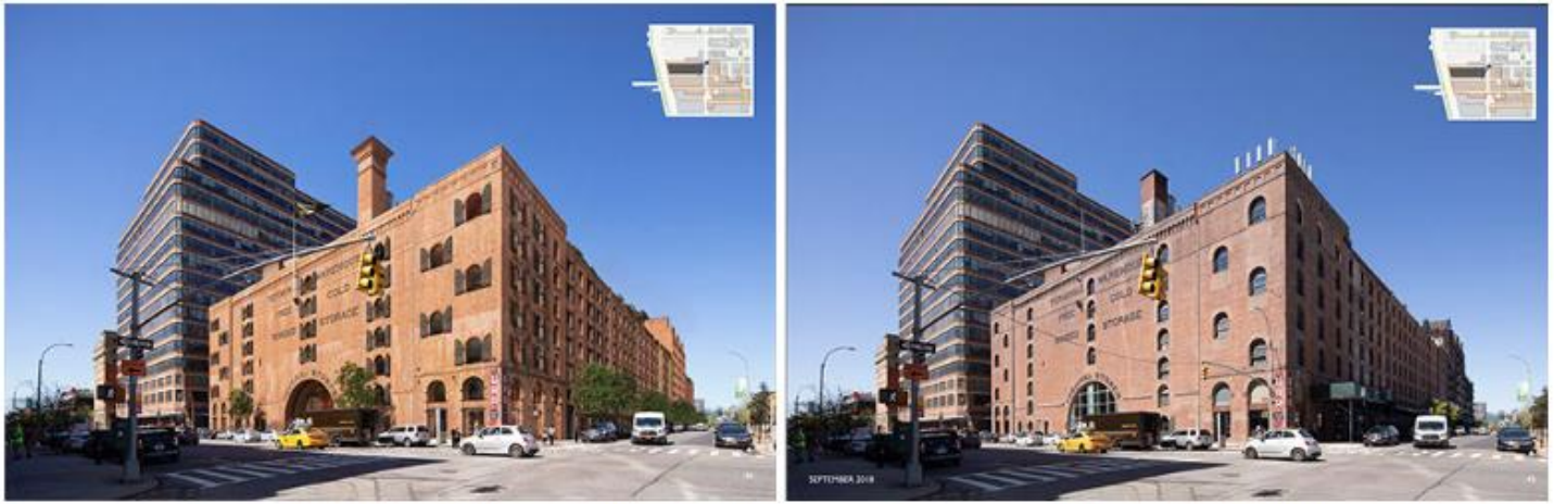
Revised rendering of Terminal Warehouse window systems (left) versus originally designed windows (right) – COOKFOX
