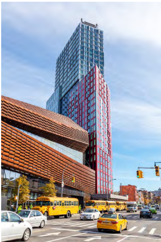
Pacific Park's first completed residential building, 461 Dean, formerly known as B2.
