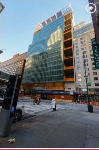
Zero Irving's construction site in Union Square. Stefano Giovannini
