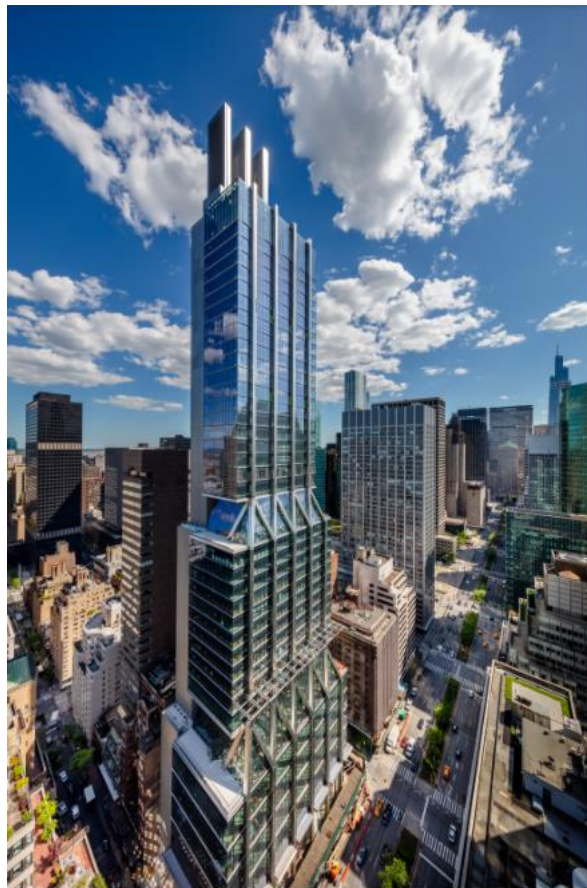
The property at 425 Park Avenue, the first full-block tower in 50 years to open on New York's Park Avenue, landed a $911.4 million refinancing loan. (Alan Schindler)
